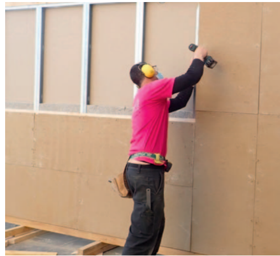
Figure 7 - Panneaux de terre extrudée - pose. © Amaco
